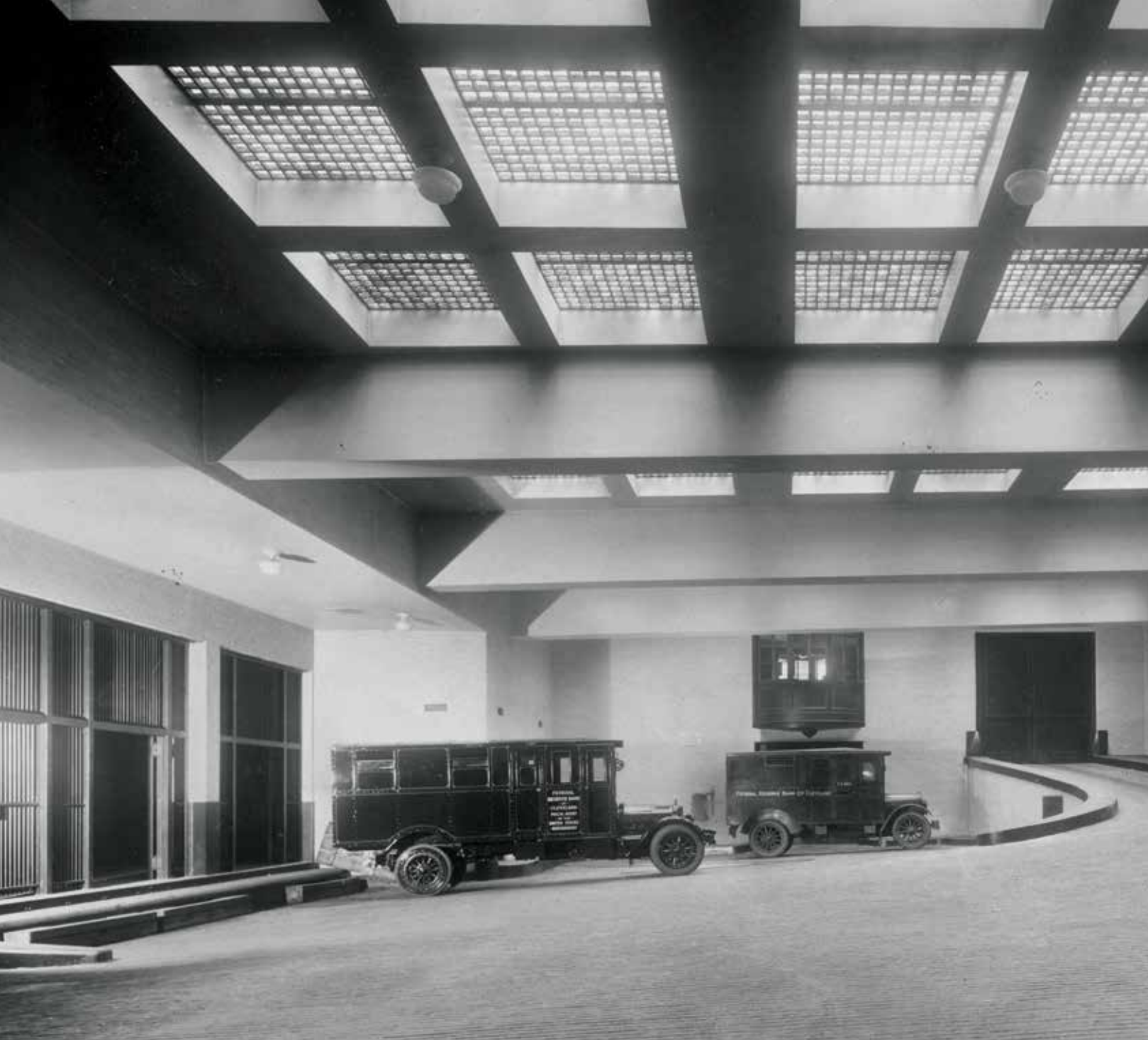
LEFT: Secure cars enter the security court entrance to pick up and drop off currency to hold in the vault, 1923. BOTTOM LEFT: Rockwell Avenue security entrance, 1923. BOTTOM RIGHT: Loading coal into the furnace to fuel the building's independent power system.
