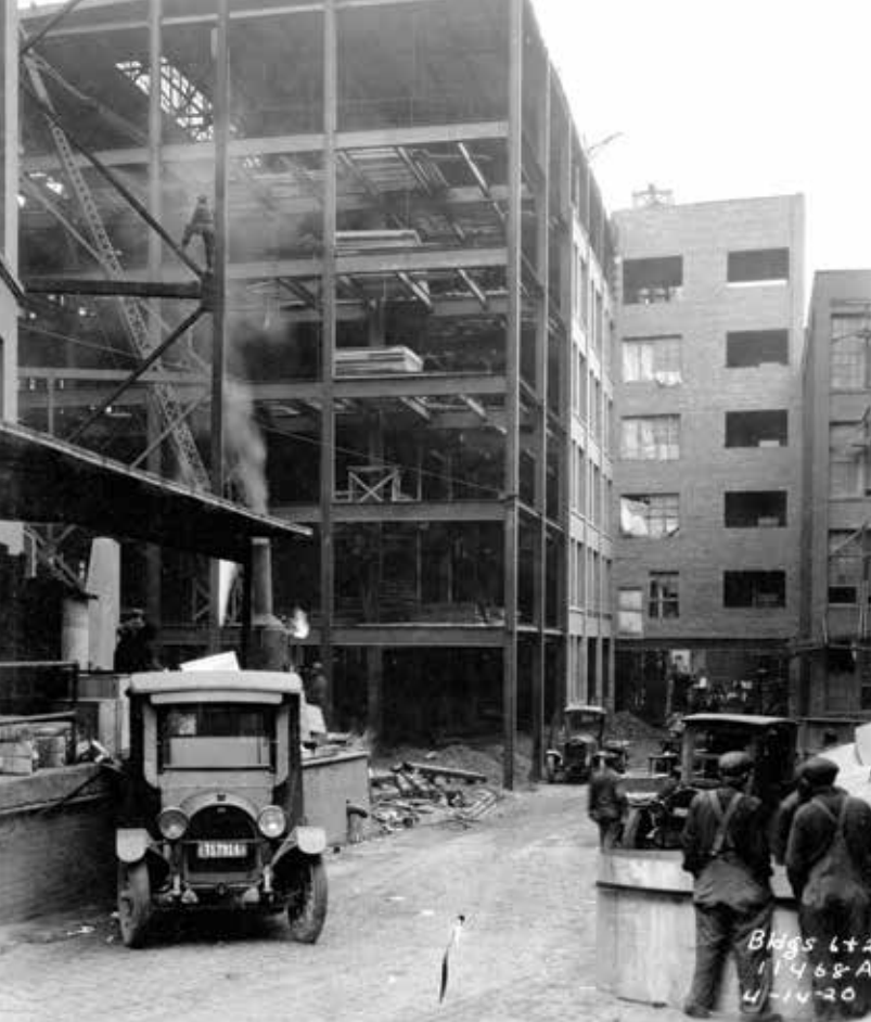
FROM LEFT TO RIGHT: The Federal Reserve Bank of Cleveland was built from the ground up using a large network of steel girders.
